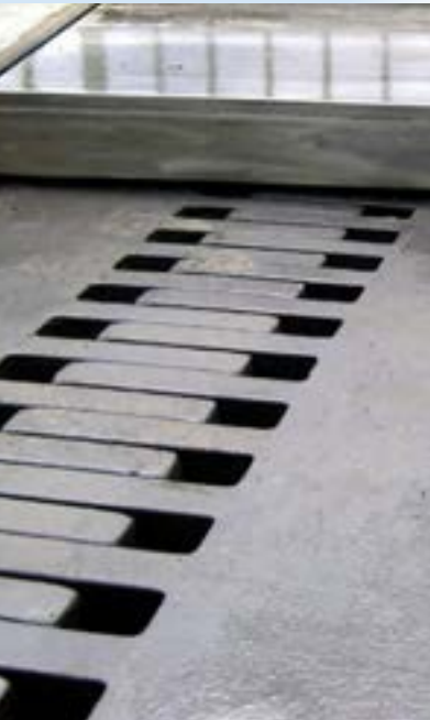
Finger expansion joint with stainless steel sidewalk
