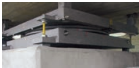
Pot bearings during installation and ...
