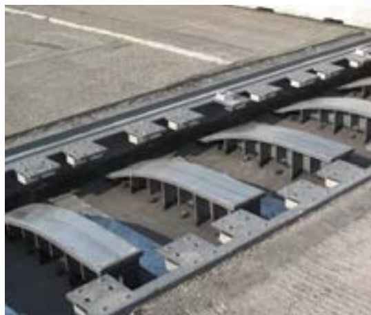
Roller shutter joint during installation
