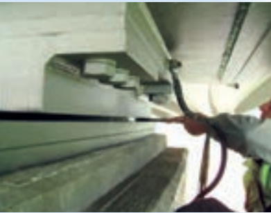
Installation of a fixed shear key
