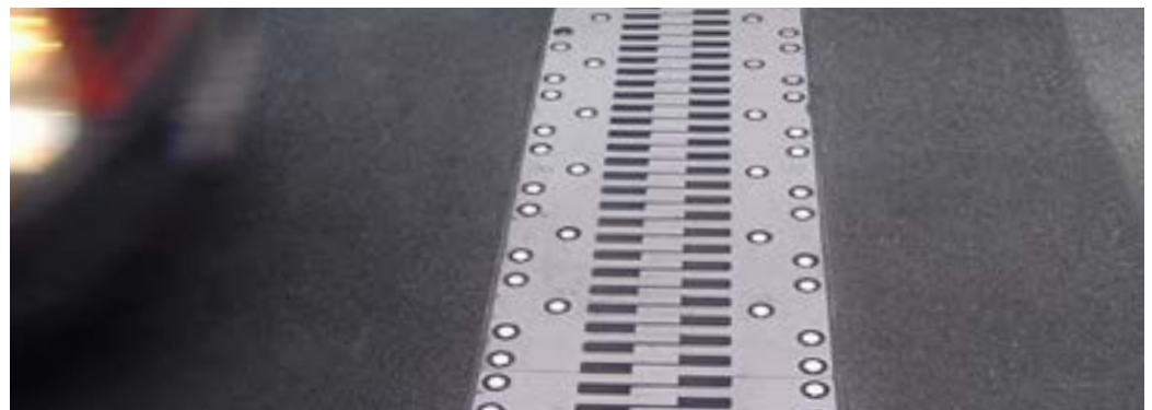
Finger expansion joint in operation
