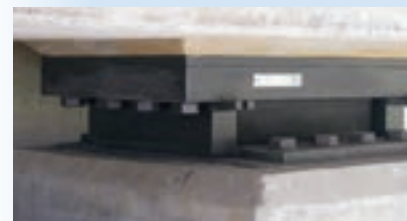
Restrained elastomeric bearing Type VS-RBU installed
