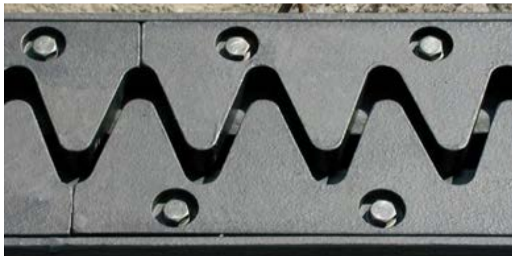
Single gap expansion joint with noise reduction installed
