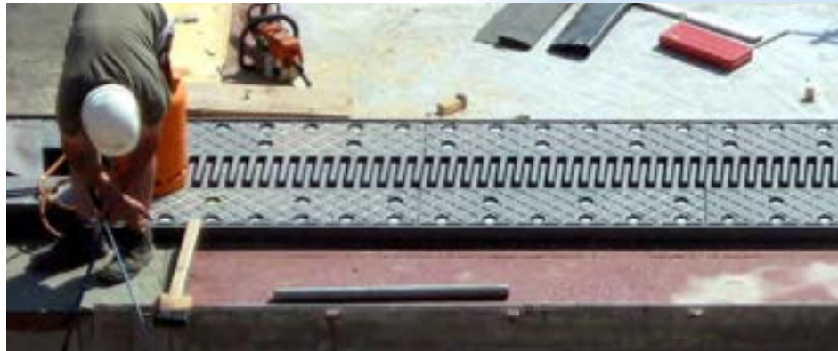
Installation of a finger expansion joint
